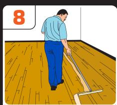
Move at a slow walk (walking too fast may produce excessive bubbling in the finish) and be sure to pour down less finish as you approach the wall.
