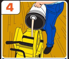
Gently mix Sport Kote® PC 128SF. Then fill a plastic watering can or the KaiMotion™ with finish. It is a good idea to fill near your starting point so any spills can be feathered into the floor
